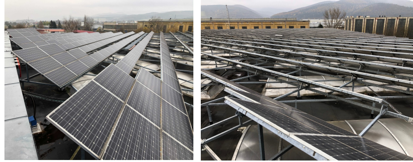
SOLAR ROOFTOP INSTALLATIONS
