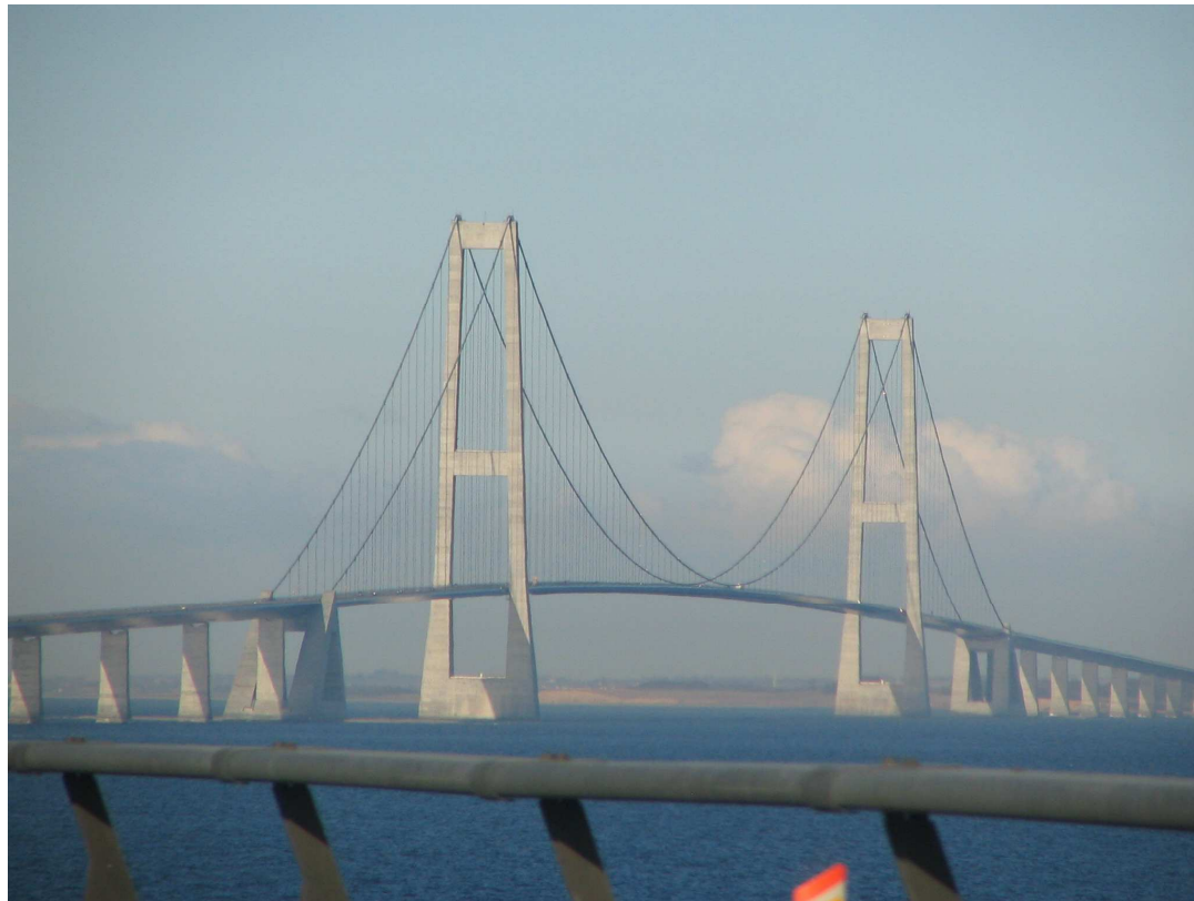
Picture Source : Bart de Witte – Big Belt Bridge - Denmark
